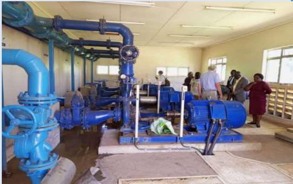
Pump house inspection at Matisi
